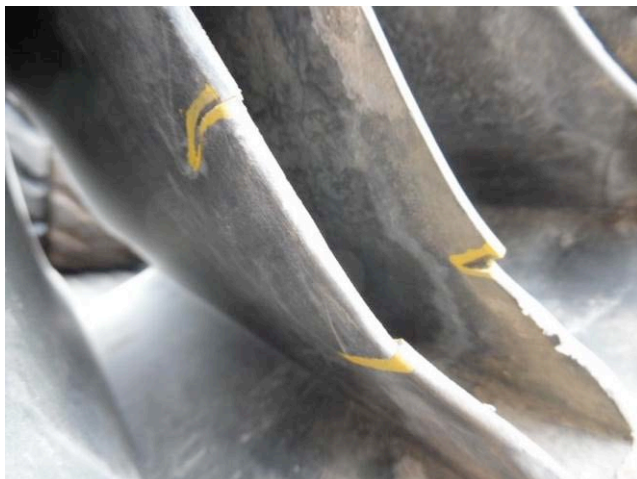
SPOKE EDGE CRACKS
